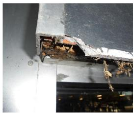
Image 11. Asbestos within wall cladding
